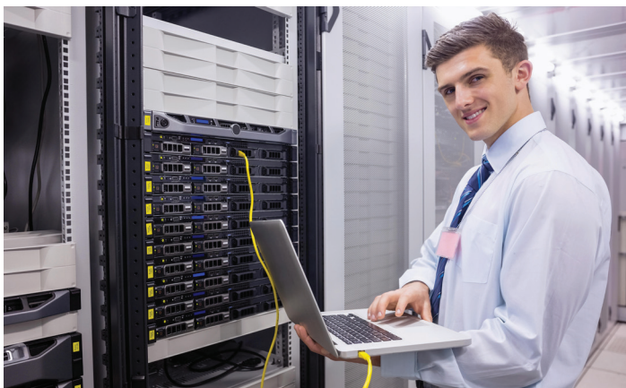
Webair Internet Development, Inc. is a cloud computing facility and data center. They received 932 kW of RNY Power in 2020.
