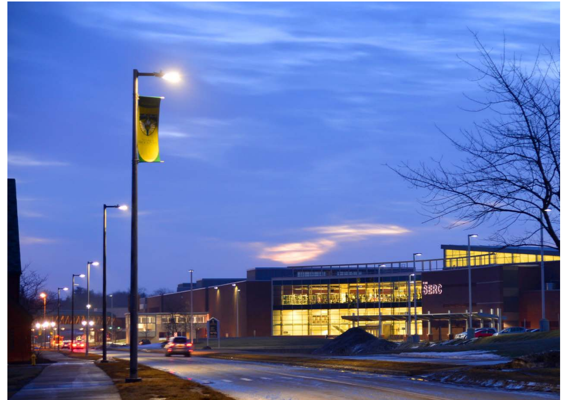
LED street lighting project completed at SUNY Brockport
