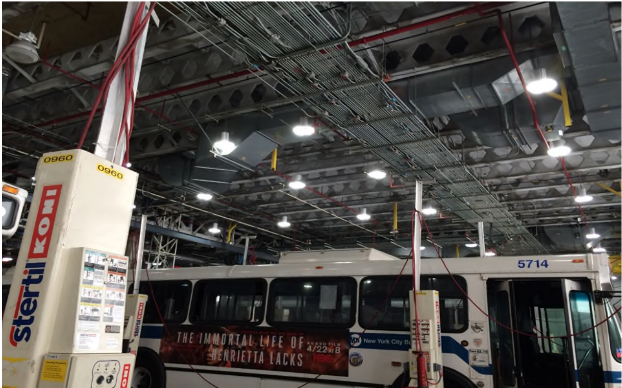
Installation of LED lighting with controls and Energy Management Systems at MTA NYC Transit Grand Ave Bus Depot & Central Maintenance Facility
