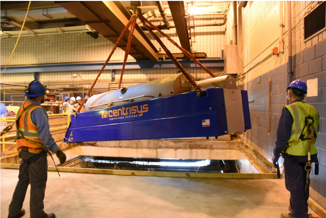
Installation of new dewatering centrifuges at NYC DEP's Hunts Point Water Resource Recovery Facility
