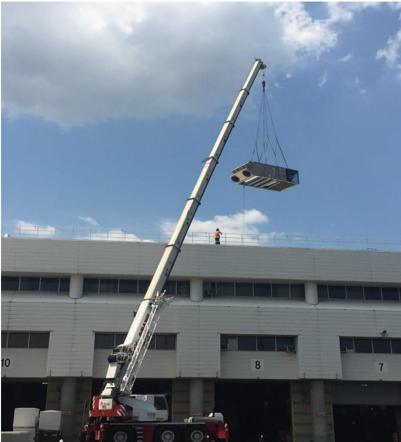
Rigging of a new high efficiency rooftop HVAC unit at LIRR Hillside Maintenance Facility
