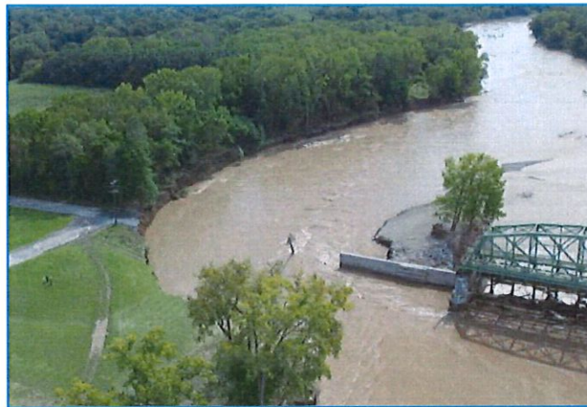
Figure 5: Lock E8 Breach after Irene and Lee
