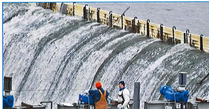
Figure 20: Flash Boards at Vischer Ferry Dam
